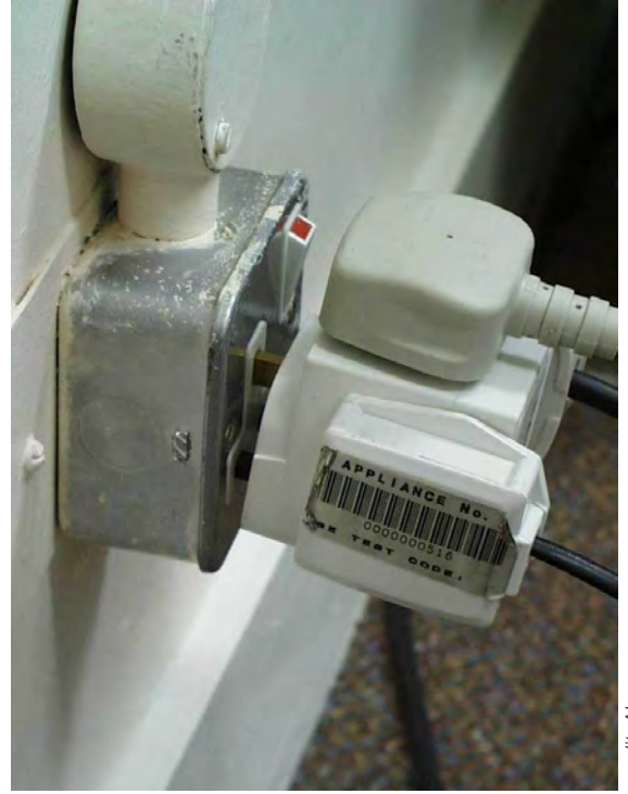
Figure 4: Mechanical loads may result in poor contact between an adaptor and a socket
